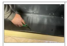
Finally once you've finished the lining, take a pair of scissors or a screwdriver and poke a few holes in the bottom where there are gaps in the wood, this is so the water doesn't build up in the bottom.
