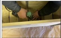
Next you want to place in the remain pieces of wood making sure the first piece has the batten screwed on.
